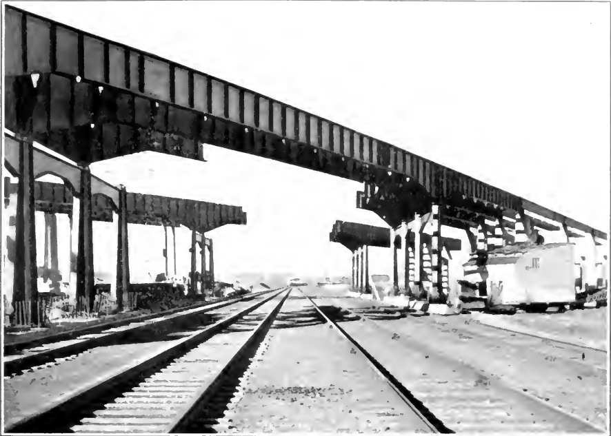
Queen Elizabeth Way — Grade Separation, C. N. R. Crossing, West of Toronto
